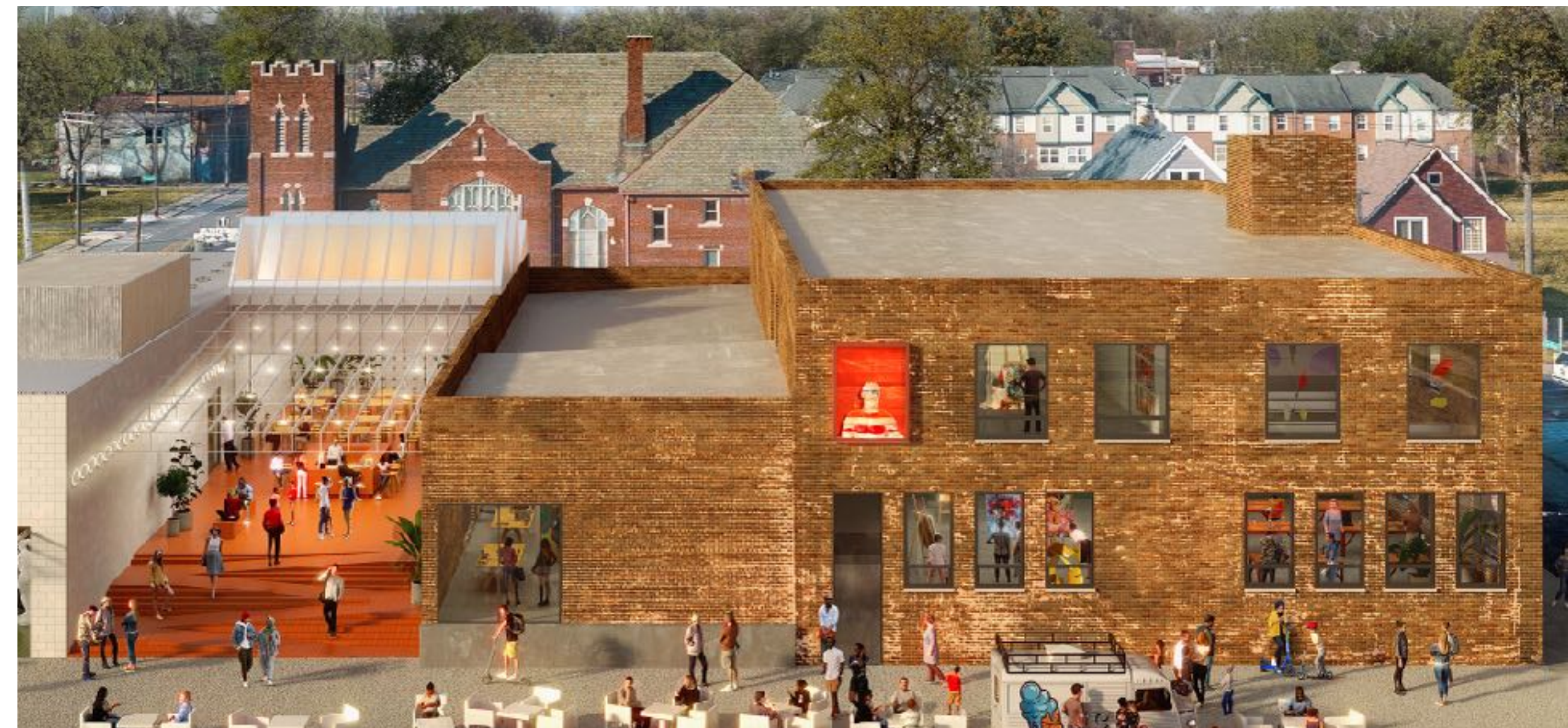
LANTERN Building, looking West, PASC gallery/studio on Bottom right
